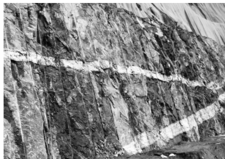
图 7 阳西片麻岩矿传统预裂爆破效果 Fig. 7 Traditional presplitting blasting effect in Yangxi
