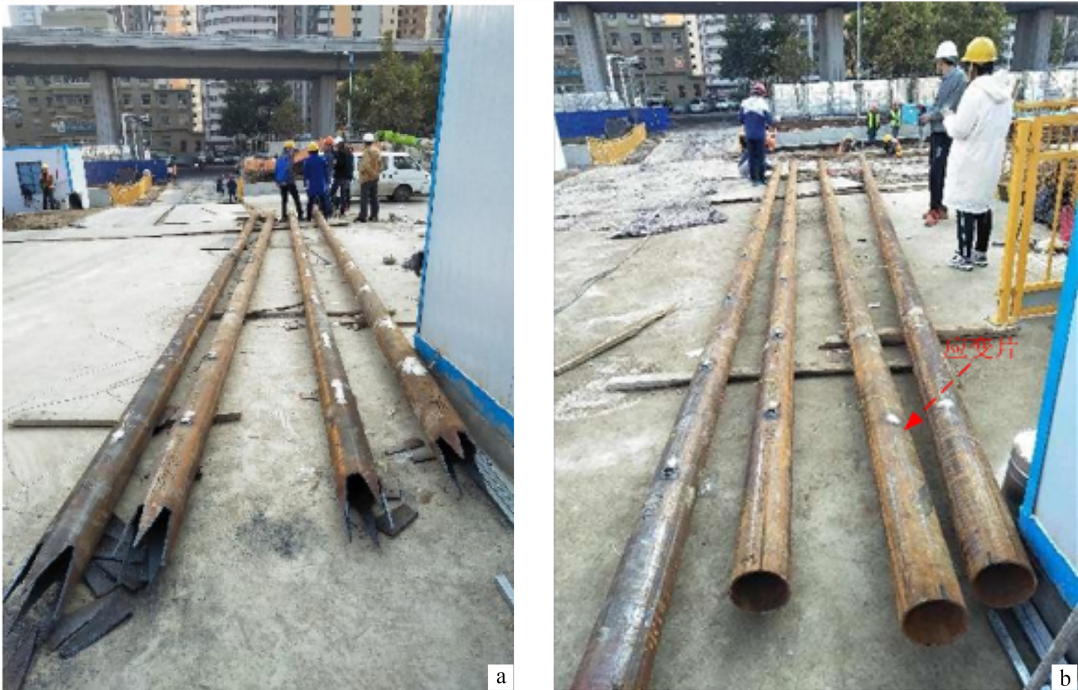
图 1 微型钢管桩(a)和应变片传感器的安装(b) Fig.1 Micro-steel pipe piles (a) and installation of strain gauge transducers (b)
