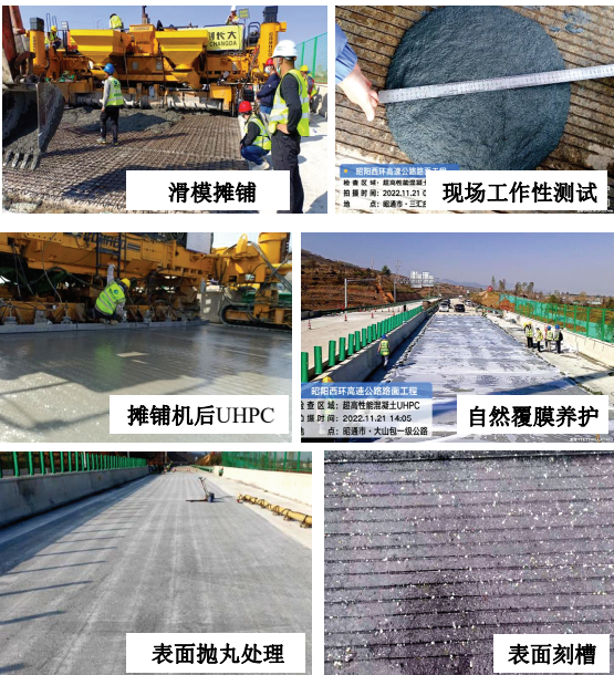
图 12 混凝土桥面含CB骨料的UHPC桥面铺装层施工过程 Fig. 12 Construction process of UHPC with CB aggregate as concrete bridge deck overlay
