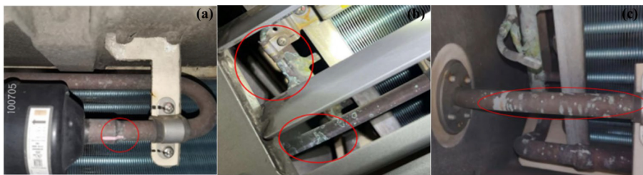
Figure 1. (a) Mild corrosion (b) Moderate corrosion (c) Severe corrosion. Source (s): Authors’ own work
