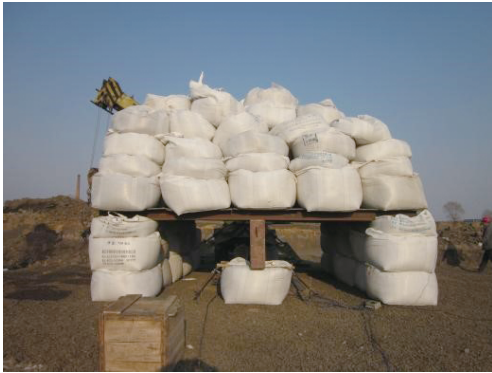
图1 现场加载装置 Fig.1 on-site loading device
