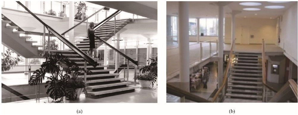
图25 大厅中央主楼梯(a)及蘑菇柱、圆形天窗(b) [12] Figure 25 The main staircase in the center of the hall (a) and mushroom columns, circular skylights (b) [12]
