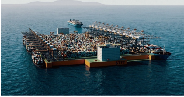
Fig. 1. Sea technology floating terminal, a floating terminal designed for large container transshipments. Reproduced from Ref. [6] with permission of Sea Technology B. Lundquist AB, ©2025.
