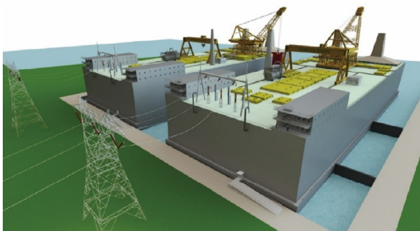
Fig. 2. Integration of Thorcon, the molten salt reactor power barge, into a shipyard-built hull, showing the floating SMR concept intended for tow-to-site deployment and seabed ballasting. Reproduced from Ref. [16] with permission of ThorCon US, Inc., ©2025.
