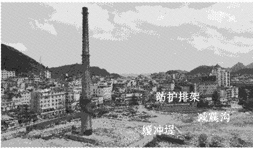
图 5 现场安全防护总体俯视图 Fig. 5 Overall top view of site safety protection
