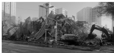
(a) 2 号楼北侧爆破效果 (a) The blasting effect on the north side of building No. 2
