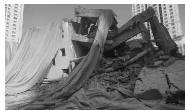
(c) 1 号楼西南侧爆破效果 (c) The blasting effect on the southwest side of building No. 1
