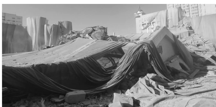
(b) 2 号楼东南侧爆破效果 (b) The blasting effect on the southeast side of Building No. 2
