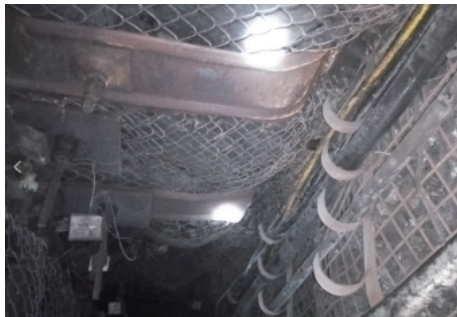
(a) 顶板切顶式下沉
