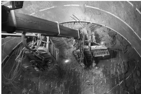
图 14 聚能管放置现场 Fig. 14 Shaped charge tube installation Site
