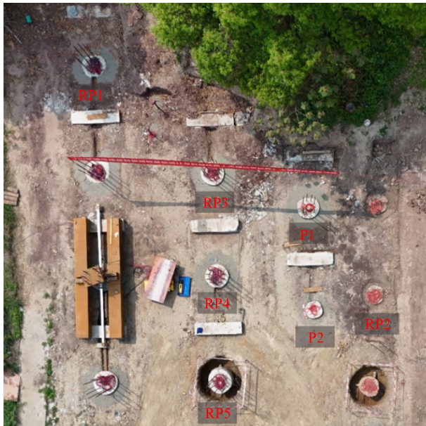
Fig. 4 Test site and layout of the test piles.
