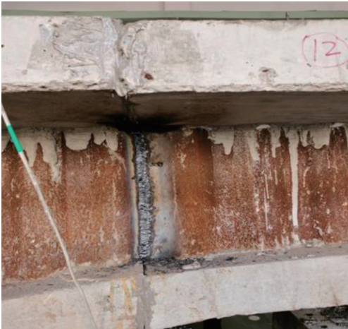
图 4 节段拼装接缝实图 Fig.4 Actual diagram of segmenting assembly joint
